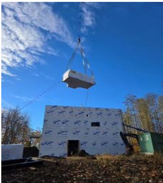
HRV Unit Lifting
