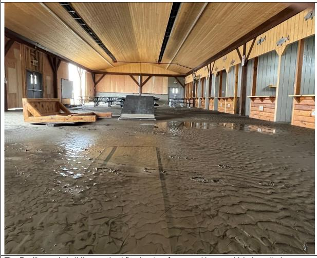
The Pavilion main building received flood waters for several hours, which deposited approximately 2" of silt throughout. The main building was assessed by the Town's insurance adjusters and it has been thoroughly cleaned via an abatement process. Wall panels and drywall and floor tiles have been removed in all booths. All remaining materials were not impacted and the building is drying until contractors return on June13th to begin repairs.
