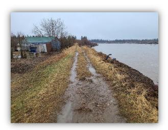
**Cleanup & Repair:** TBD. Further observation in the coming months will provide a basis for repair. If the berm continues to worsen, a geotechnical assessment is recommended to assess the cohesion and saturation limits of the berm's material.
