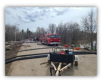
**Cleanup & Repairs:** Hundreds of hours of labour and pumping from internal and contracted services/ equipment were required to clear water from the ravine and allow access to the lift station (pictured above). Cleanup required will involve removal of debris and road materials from ditches and placement of a new granular base.
