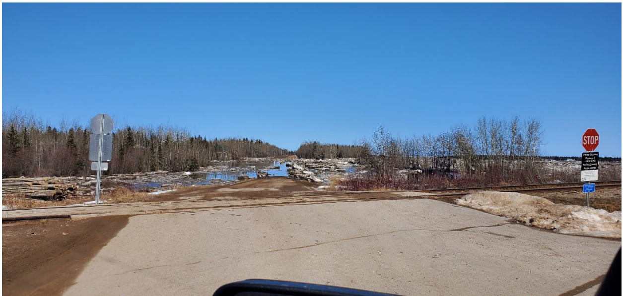
Water Treatment Plant Road – May 5, 2022
