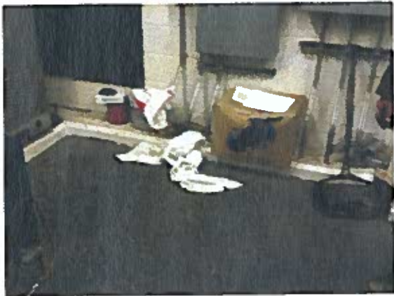
Boxes being stored in Mechanical room
