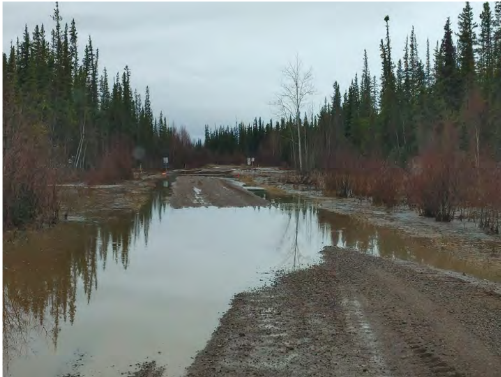
Figure 27: Water Treatment Plant Road - May 10
