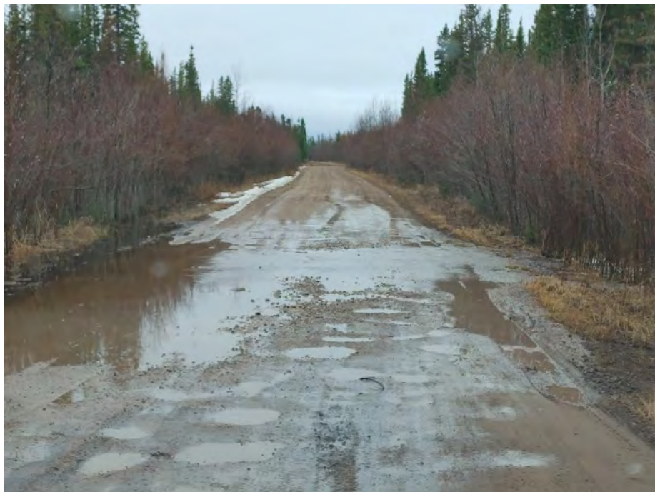
Figure 32: Water Treatment Plant Road - May 10
