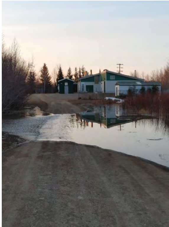
Figure 20: Water Treatment Plant Access - May 6
