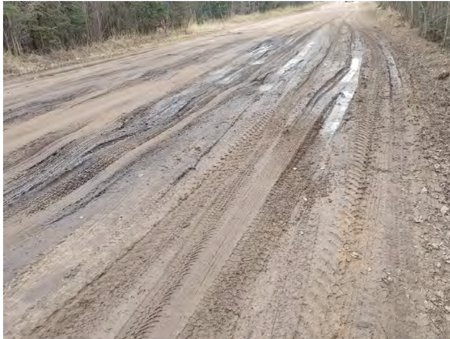
Figure 34: Lagoon Road – May 20
