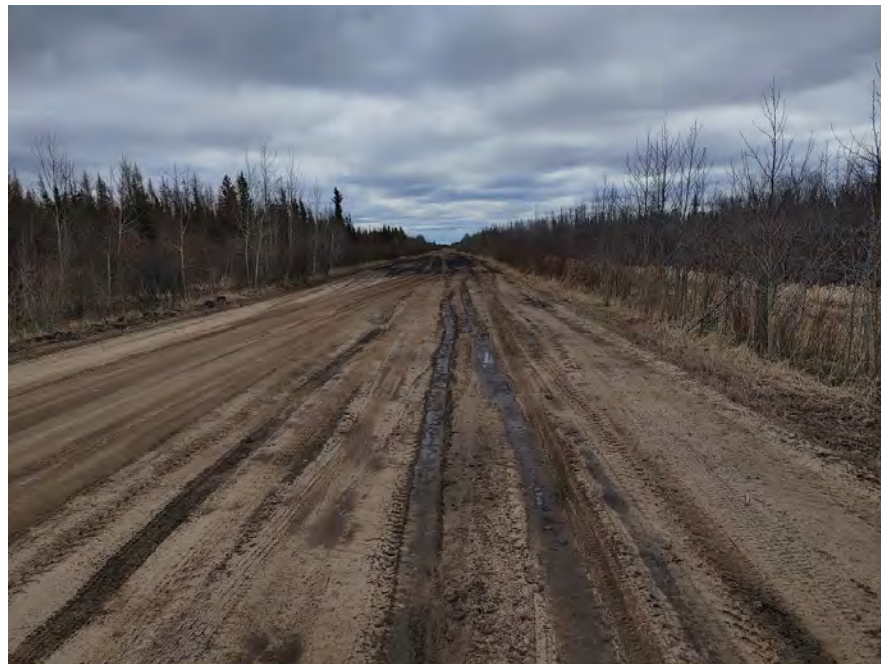
Figure 35: Lagoon Road - May 20
