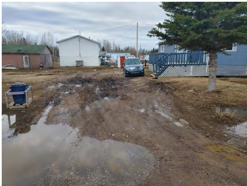
Figure 15: Back Road Driveway Damage
