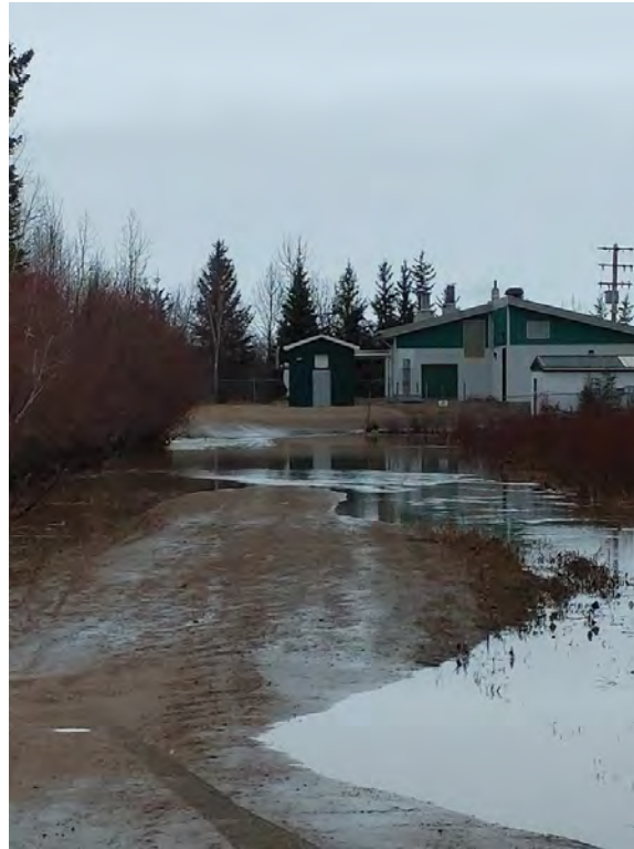
Figure 22: Water Treatment Plant Access - May 10
