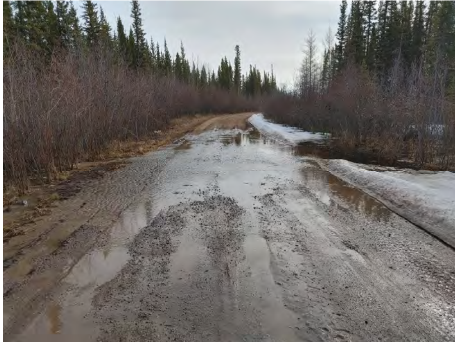
Figure 31: Water Treatment Plant Road - May 7
