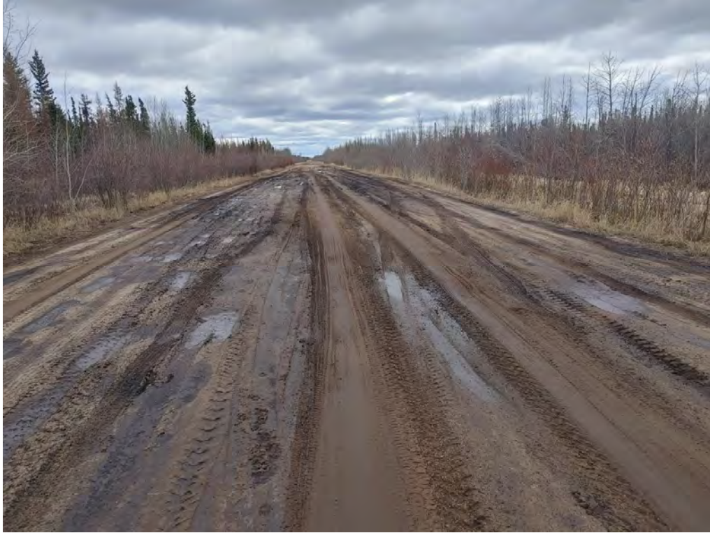
Figure 36: Lagoon Road - May 20
