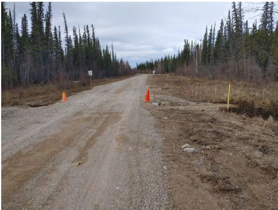
Figure 29: Water Treatment Plant Road - Additional Culvert - May 20
