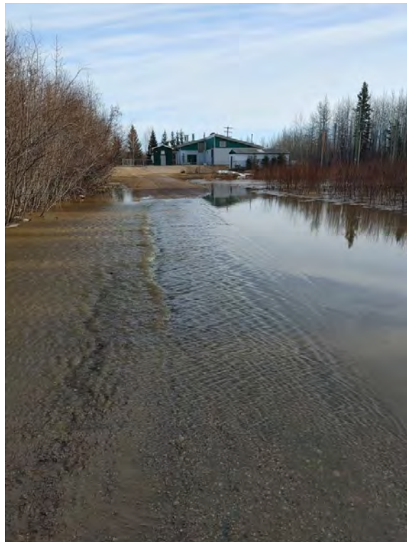
Figure 21: Water Treatment Plant Access - May 7
