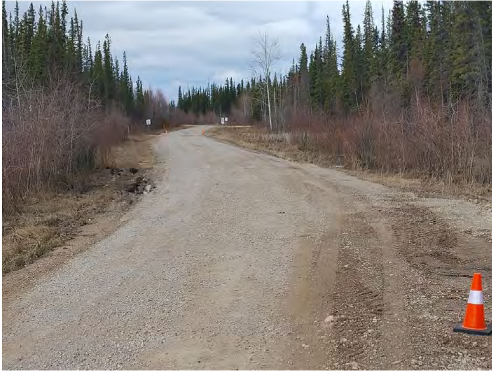
Figure 28: Water Treatment Plant Road - May 20
