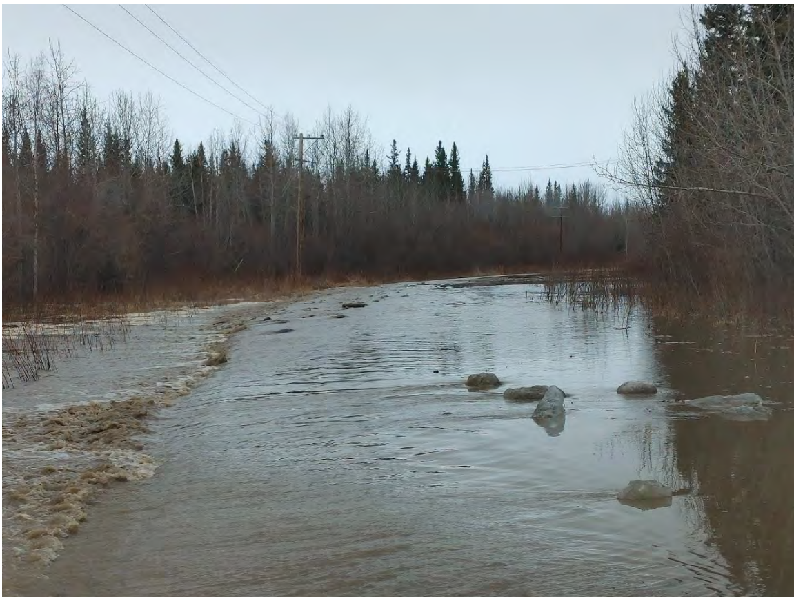
Figure 16: Water Treatment Plant Road - May 10
