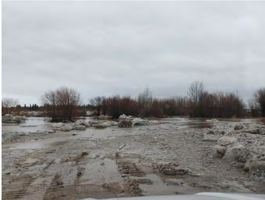
Figure 17: Water Treatment Plant Road - May 10
