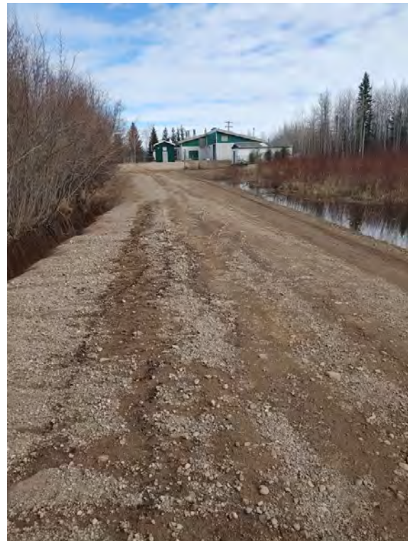
Figure 23: Water Treatment Plant Access - May 20
