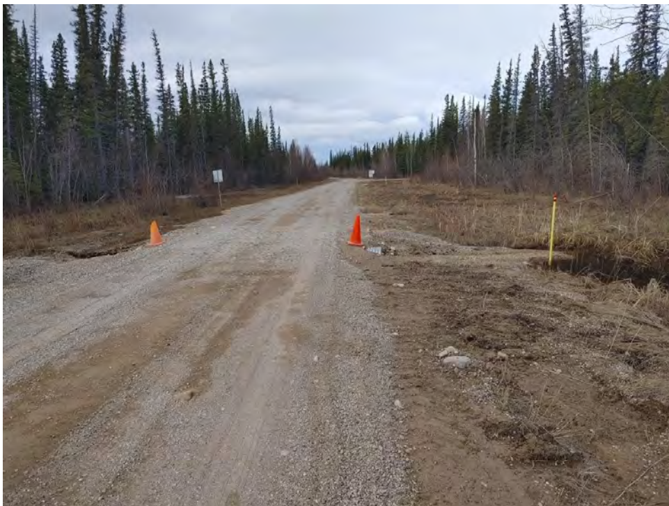
Figure 29: Water Treatment Plant Road - Additional Culvert - May 20
