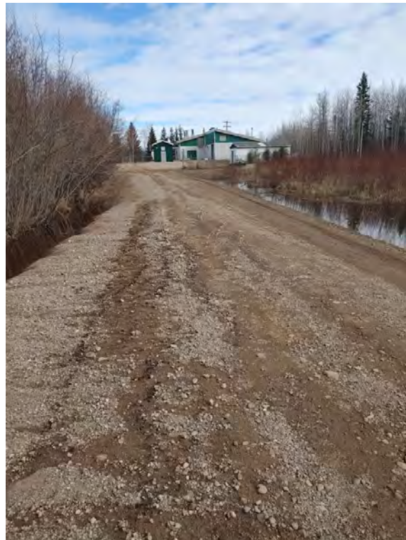
Figure 23: Water Treatment Plant Access - May 20
