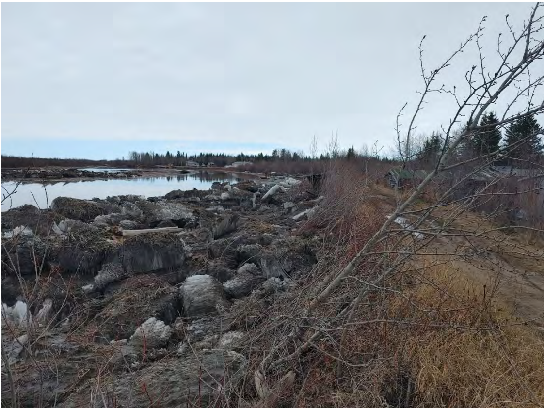
Figure 11: Ice Along Berm - May 20
