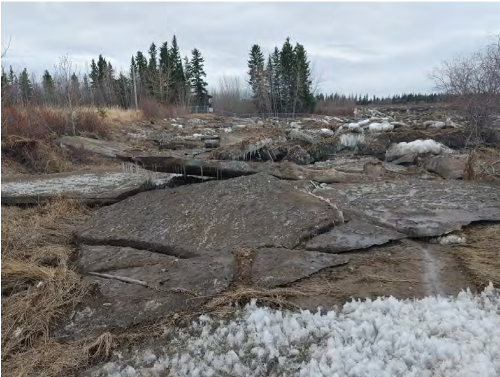
Figure 13: Ice Along Berm - May 20
