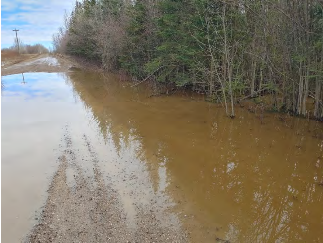
Figure 19: Water Treatment Plant Road Ditch - May 20
