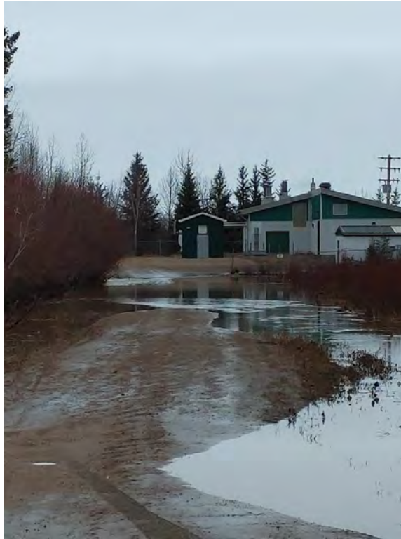
Figure 22: Water Treatment Plant Access - May 10
