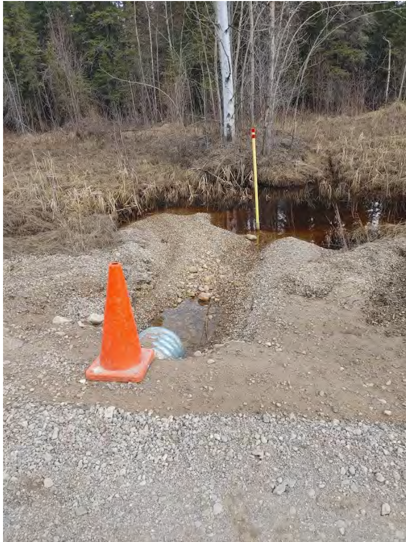
Figure 30: Water Treatment Plant Road - Additional Culvert - May 20
